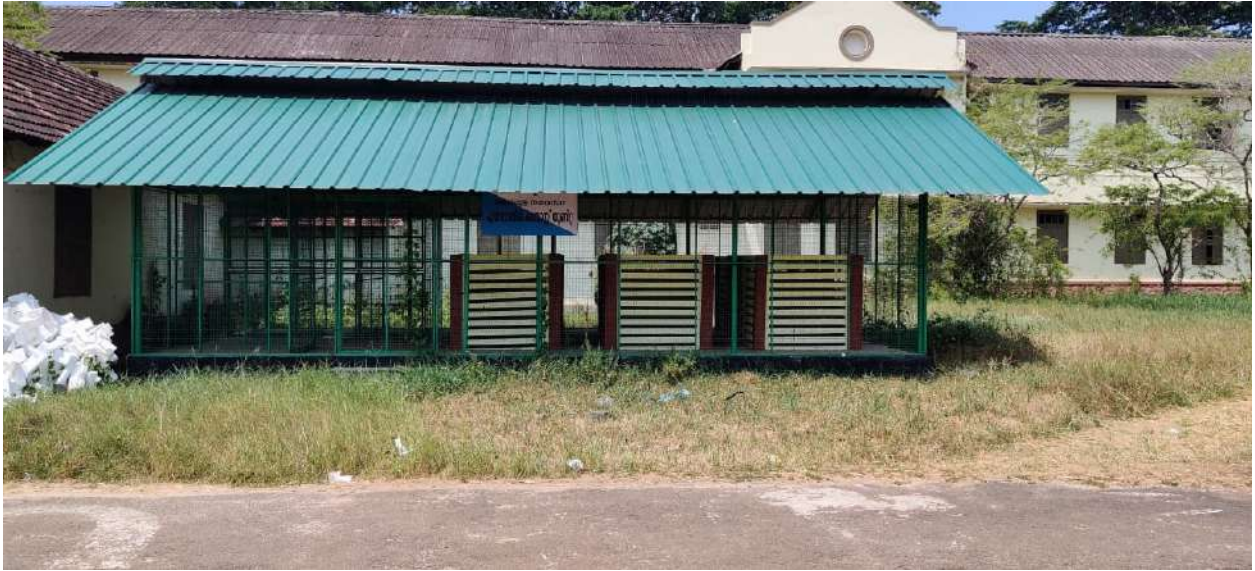
Waste segregation Unit
